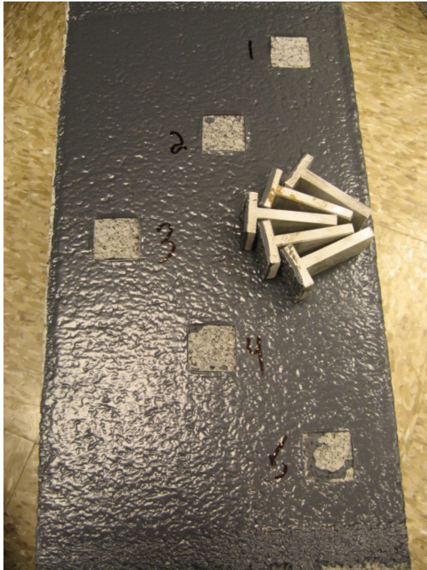
Photo No. 3 Pull-Off Strength - CMU Substrate All Results
